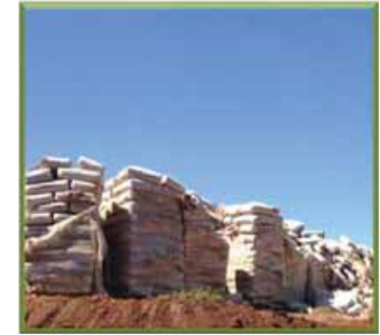
Picture 18: Cement packets exposed to the weather
