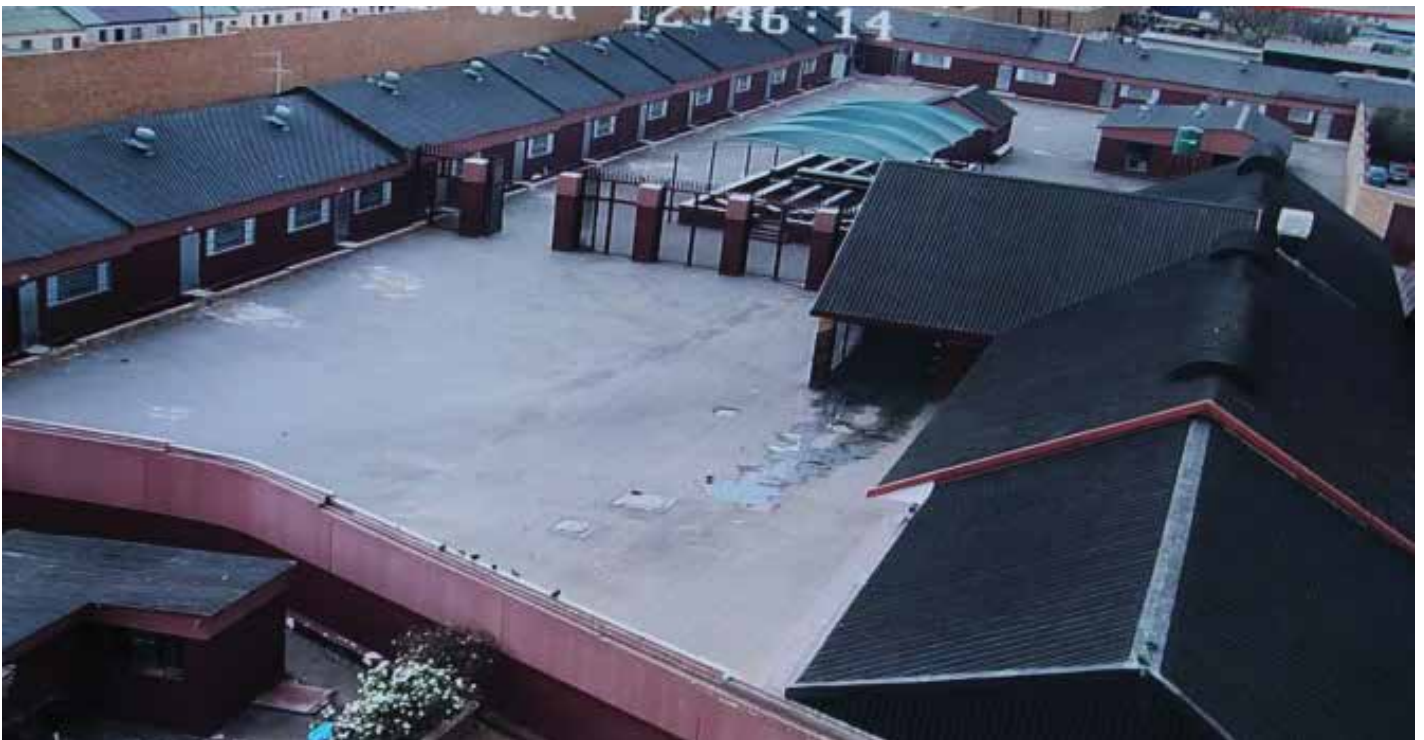
Picture 1: The holding facility that was not optimally used
