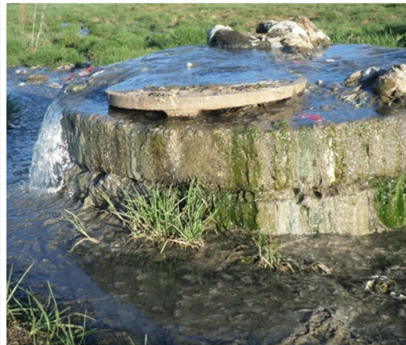
Phuthaditjhaba wastewater treatment works is non-functional due to serious vandalism, resulting in sewage overflows in the area (Maluti-A-Phofung, Free State)
