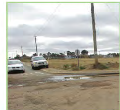
Picture 26: Ponding water
