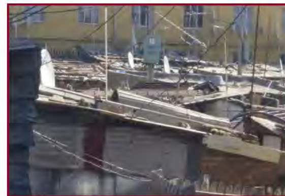
Picture 1 shows congestion and numerous electrical connections.
