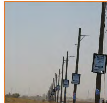
Picture 17: Poles without light fittings
