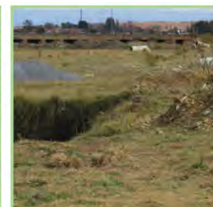
Picture 31: Exposed excavation
