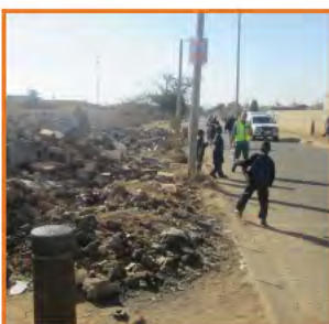
Picture 14: Destroyed multi-purpose centre
