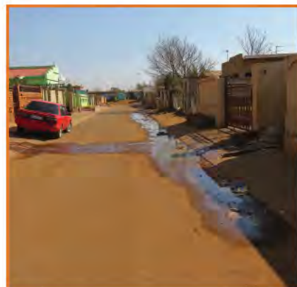
Picture 19: Raw sewage flowing into street
