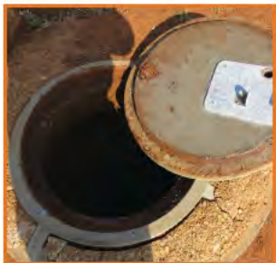
Picture 10: Cracks on the concrete apron
