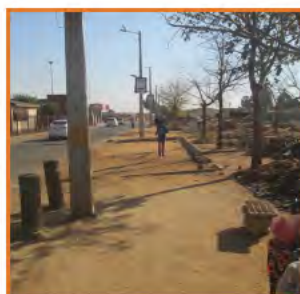
Picture 15: Section of missing paving
