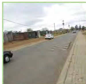
Picture 29: Vegetation growth on sidewalk
