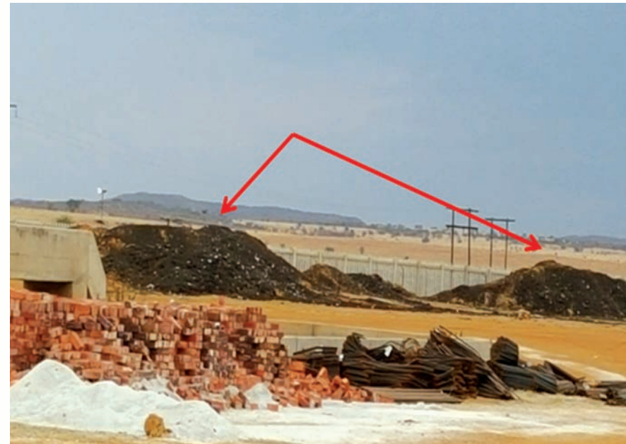
Picture 8: Dried sludge (by-product) not disposed of accumulating on site at the existing Maquassi WWTW
