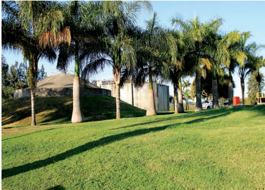
Picture 9: Good condition of the Tzaneen WWTW
