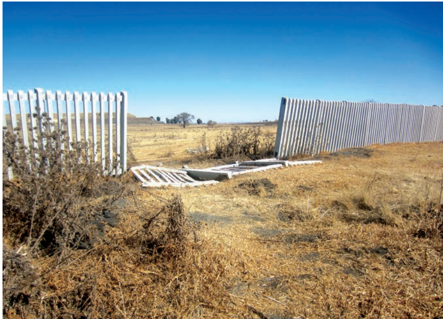
Picture 3: Damaged palisade fence around the Evander WWTW
