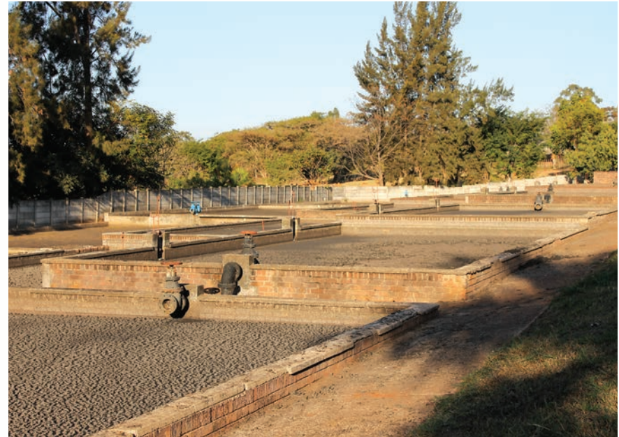
Picture 10: Condition of the infrastructure
