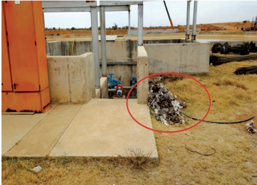
Picture 1: Filtered waste material that was not disposed of and was left exposed on site (NW)
