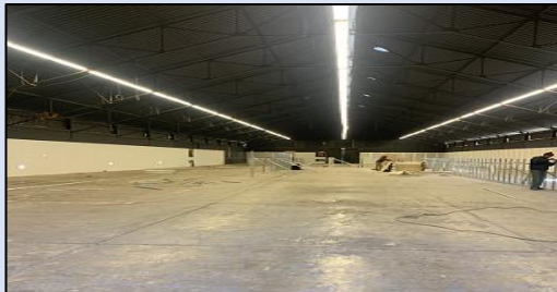
Drywall installation in progress
