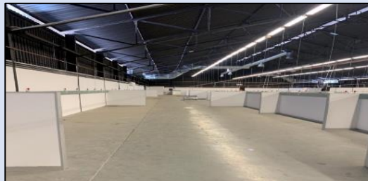
Progress on hall preparation
