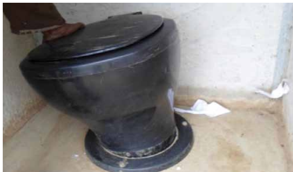
Picture 4: Toilet ring loosely fitted
