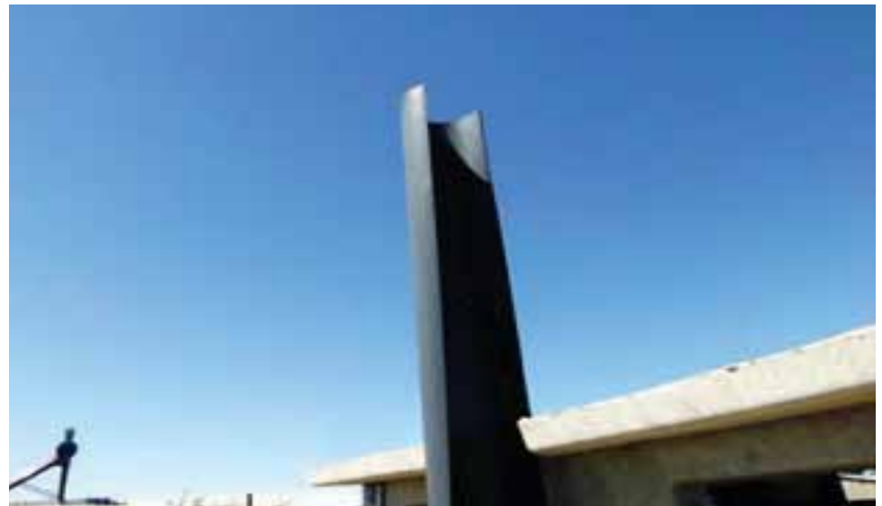
Picture 2: Vent pipe broken
